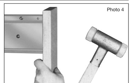
Ensure perfectly closed joint by using wooden block and hammer from the blank end of the second Powerail section. Attach joint fish plates and tighten properly.
